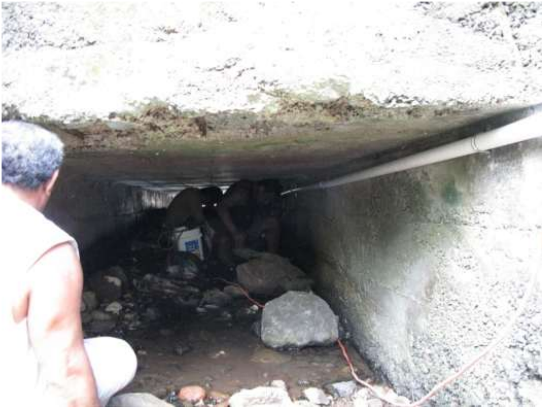
Village helpers installing intake line through culvert under the road.
